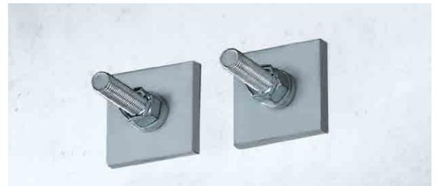
Rear-side anchoring of the support console to the reinforced concrete beam.
