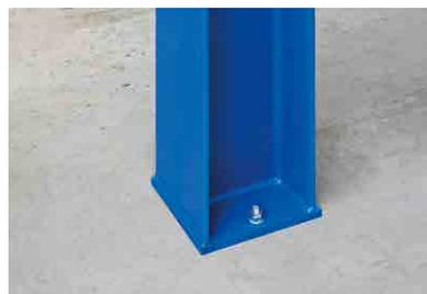
Rigid portal structures allow small pillar bases, which are secured using dowels.
